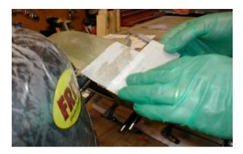
The extra resin from the cloth will be absorbed into the peal-ply and will hold it in place for later removal.
