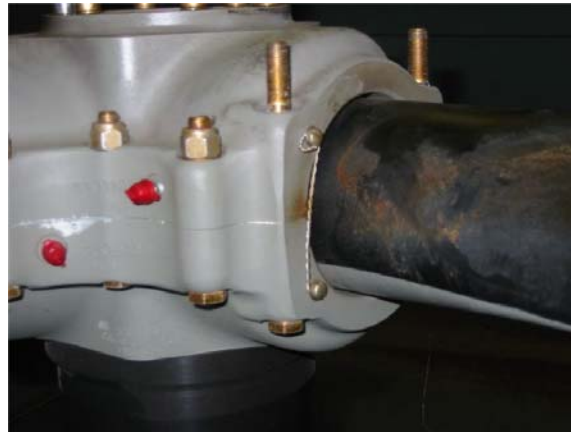
FIGURE 2-1. Grease Leak Residues
